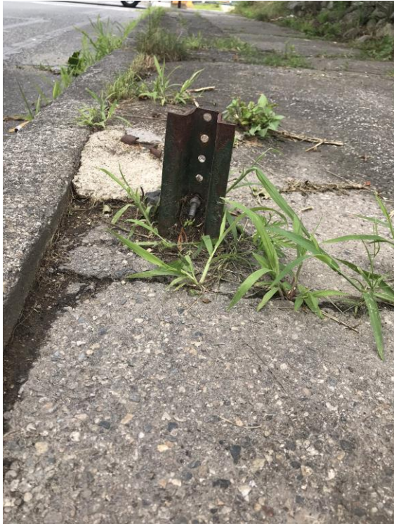
Tripping hazard on sidewalk (on Apsley Street by Lincoln Street intersection)
