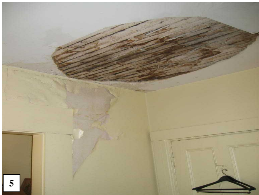
Before: 4. Ceramics class taking place in deteriorated basement. No ADA accessibility. 5. Deteriorated plaster ceilings 6. & 7. World's oldest chairlift is only ADA accessibility to second floor. Third floor is not used.
