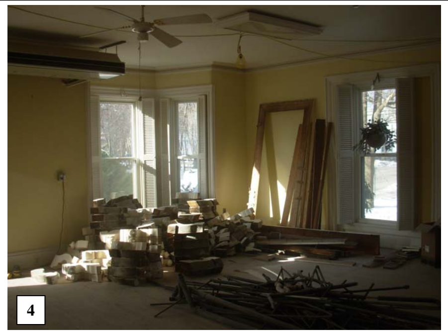
During: 1. Removal of aluminum siding reveals lost quoins 2. - 4. Removal of woodwork, doors & brackets for reuse & reinstallation
