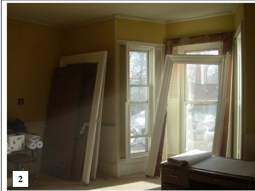
During: 1. Removal of aluminum siding reveals lost quoins 2. - 4. Removal of woodwork, doors & brackets for reuse & reinstallation
