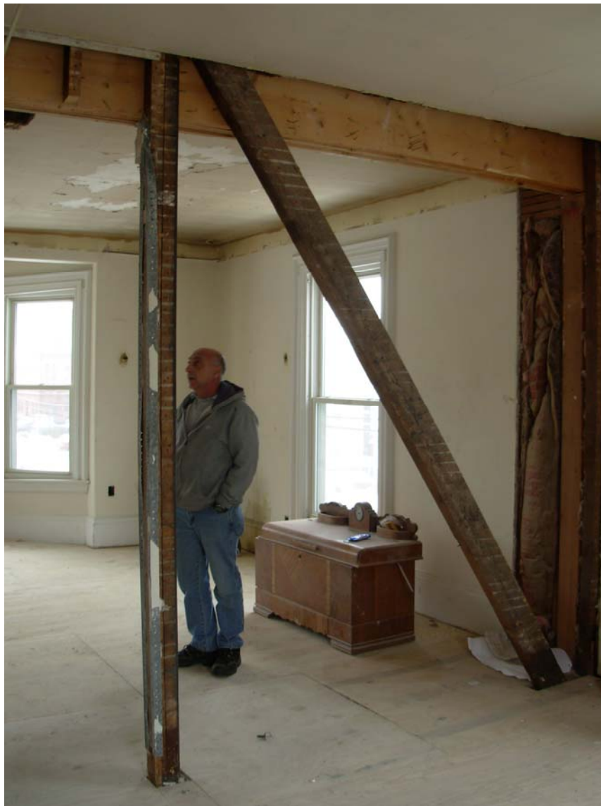
Tie rod hidden inside wall dividing craft room.
