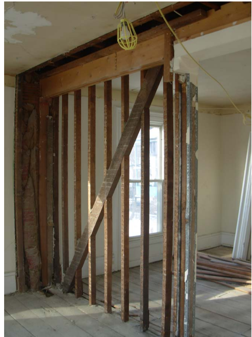
Tie rod hidden inside wall dividing craft room.
