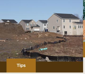
Straw wattles should not be used alone as they degrade too quickly. Use straw wattles with silt fence. Also do not stake through them as it rips through the netting. Instead, stake them in an upside down "V".
