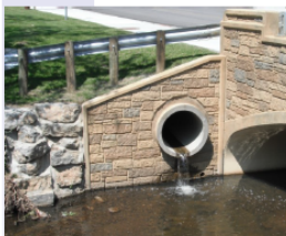
Outfall-rainwater into stream
