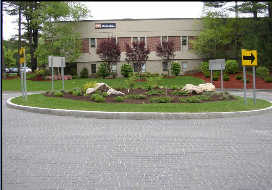
STAMPED COLORED PAVEMENT FOR TRUCK APRON
