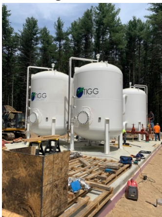
Carbon filter vessels at Cranberry Well
