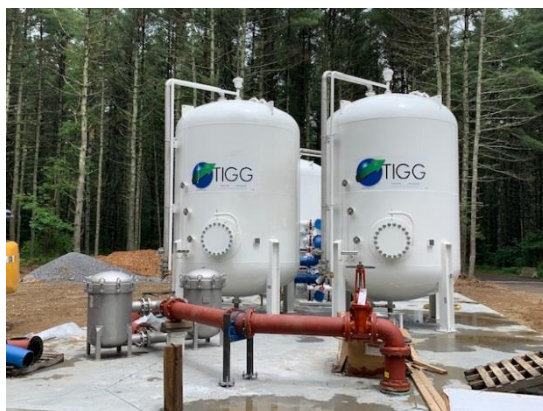
Carbon filter vessels at Cranberry Well
